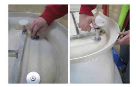
6. Use the levelers on the pedestal to make any needed height adjustments.
